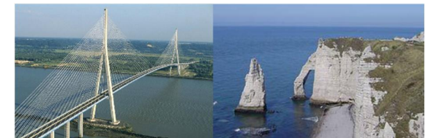
Normandy Bridge (left); Manneporte Arche in Etretat
